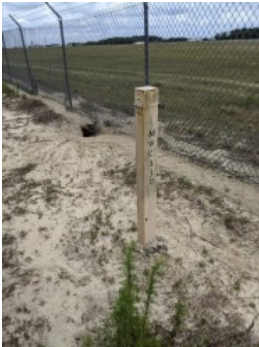
Photo 21 Monitoring well for reclaimed water use.
