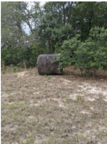
Photo 11 Concrete culvert, Parcel 4.
