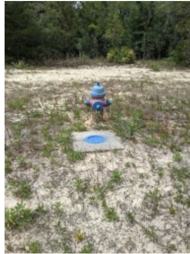
Photo 26 Parcel 1, fire hydrant and water shut-off.
