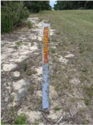
Photo 19 Reuse water line marker, Parcel 2.
